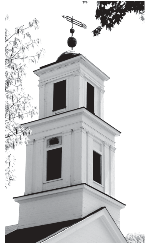
Marlborough Congregational Church parishioners are working to restore the historic church steeple.
