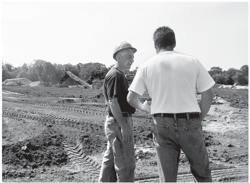
Parks and Recreation Director Rich Calarco (in the hard hat) speaks with a contractor from Simscroft-Echo Farms at the future home of the five-field athletic complex along East Street. Calarco said this week the project is running on-time and within budget and expects a fall 2009 opening.
