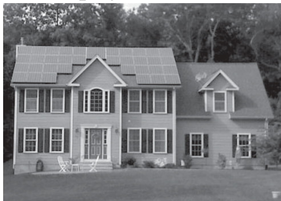
Pictured above is Travis and Michelle Cohen's home at 91 Cirillo Dr. with its new addition of 36 solar panels. The Cohens will host an open house tomorrow from 10 a.m. to 4 p.m. for neighbors to come and view their panels as part of the third annual Solar Tour. The Cohens' home is one of two Colchester residences participating in the tour.
