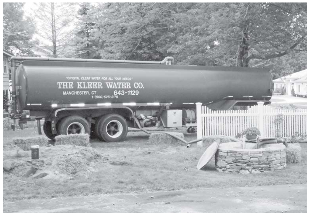
A dug well at a residence on School Drive ran dry in early September, but there are different opinions as to the cause. Pictured is a water tanker hooked up to the dug well, right, and the new drilled well, left.
