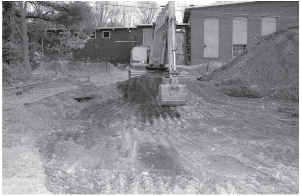
Interim cleanup at a town-owned industrial building on Watrous Street is complete, the Brownfields Redevelopment Agency announced this week. Shown here is a backhoe removing contaminated soil at the site.
