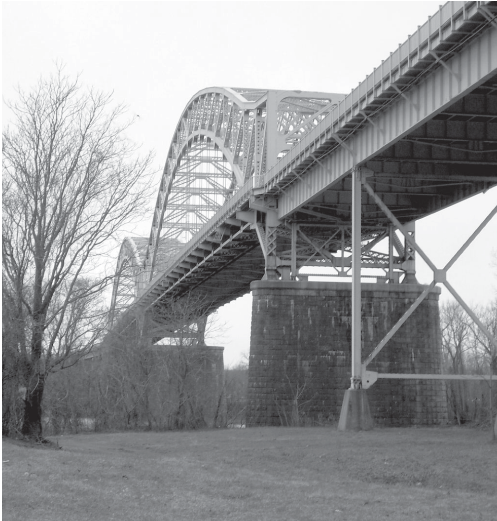
The Middlesex Chamber of Commerce recently discussed plans to revamp the Arrigoni Bridge. Repairs will begin this summer and the final stage is slated to finish in October of next year.
