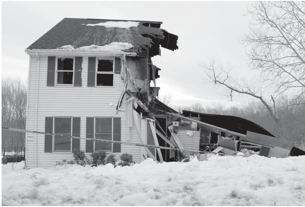
The propane explosion on Jan. 29, 2011 destroyed a duplex on Summer Street in Portland. No ignition source was ever found.
