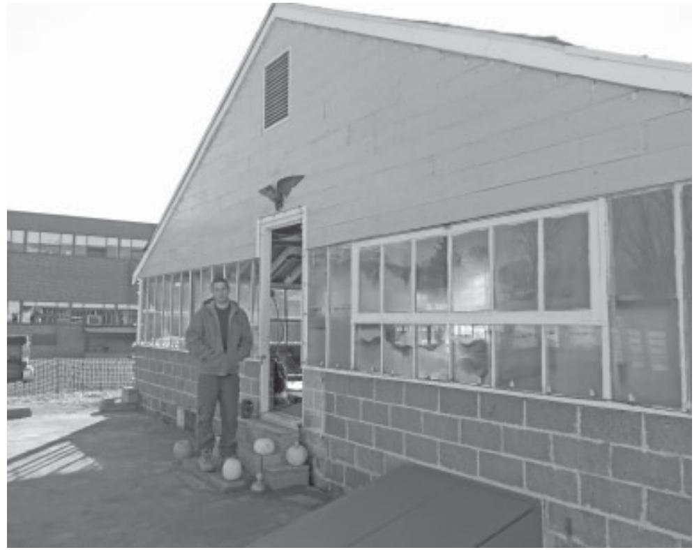
The revitalization of the former Geato’s Greenhouse and Flower Shop is the feverish work of Chris Cusack, who plans to turn the property into Alchemy Greenhouses . The new business will specialize in aquaponics, a system that raises marine animals and plants and herbs. Cusack has already revamped the former storefront of the greenhouse, which is located at 12 Middlesex Ave.
