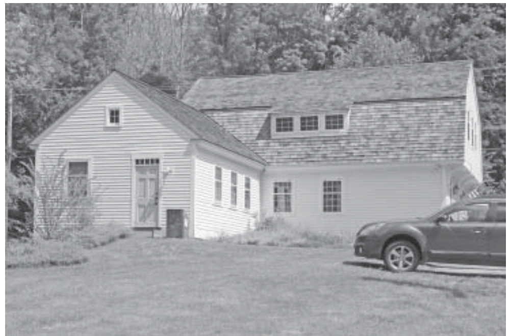
A petition against a proposed addition to Middle Haddam Public Library has generated nearly 100 signatures.
