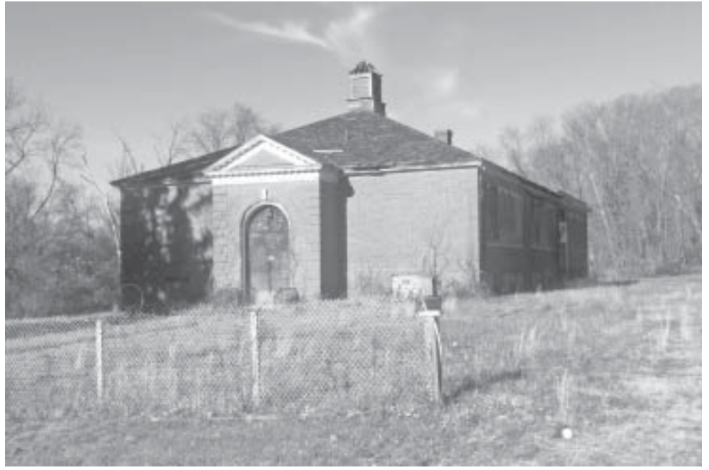
The old schoolhouse on the edge of the Middle Haddam Historic District is ticketed for possible demolition in the spring – a message that caught members of the Town Council by surprise last week.
