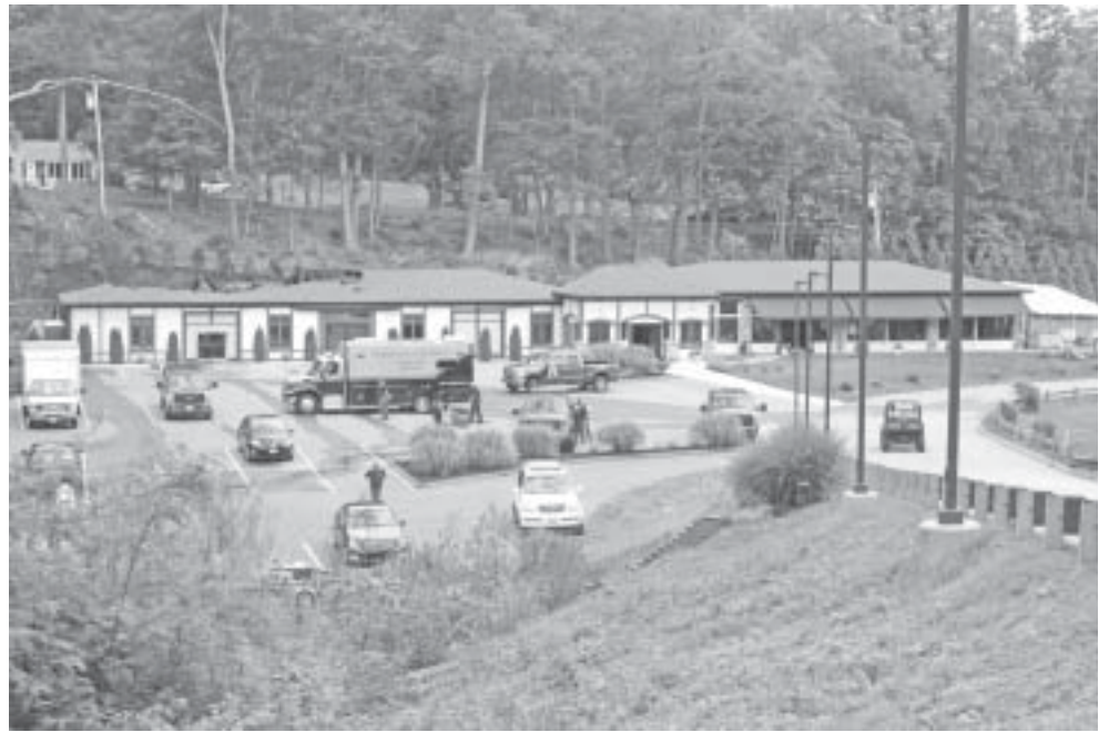
A fire at a clubhouse on the East Hampton side of the Saint Clements Castle and Marina was accidental, according to a report from the East Hampton fire marshal’s office released more than three months later. No fire code violations have yet been identified at the facility that officials say was operating without the appropriate permits and food service licenses.
