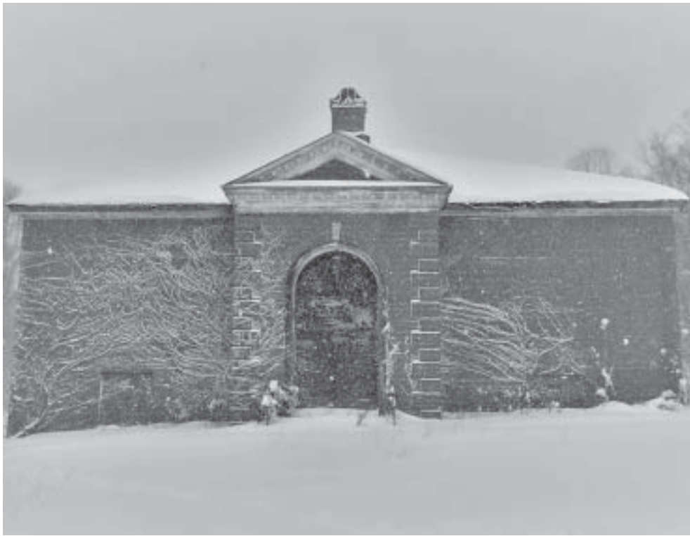
The Middle Haddam Association, the struggling nonprofit organization that purchased the Middle Haddam School over a decade ago to prevent it from being converted into condominiums, is asking for the town's help to save the building from demolition. Photo from the Friends of the Middle Haddam School Facebook page.
