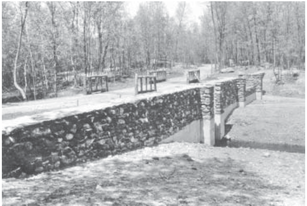
As part of the CCC’s nature conservation movement, members from Camp Stuart in East Hampton built the stone and concrete dam at Day Pond State Park in Colchester.
