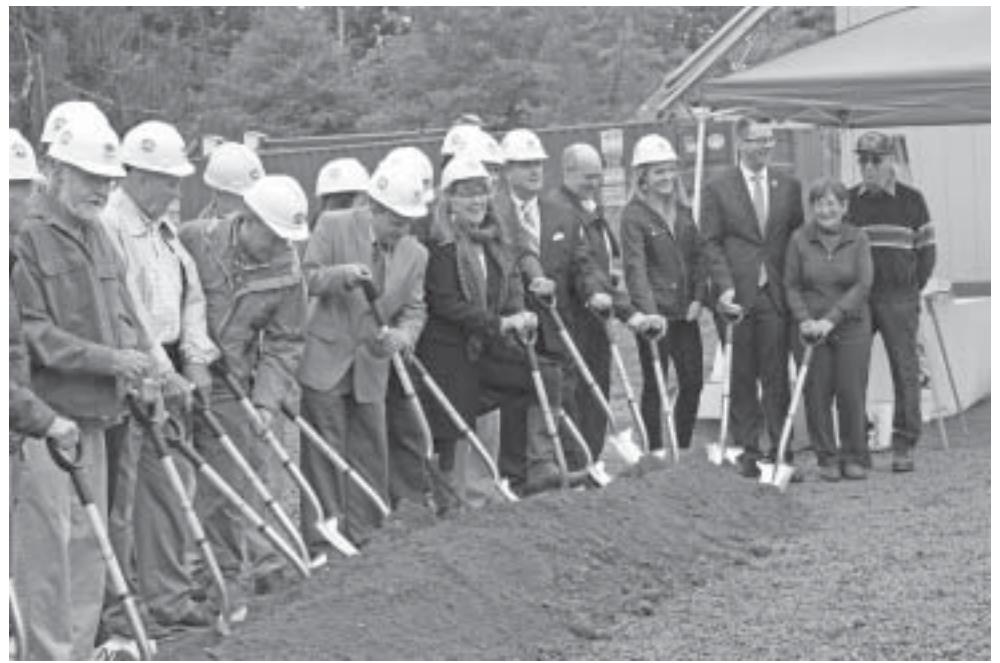
An array of those responsible for the new municipal hub to be constructed on Route 66 assembled last Friday to break ground on the $18.98 million project. The 33,400-square-foot building will include town hall offices, the police department and the Board of Education.
