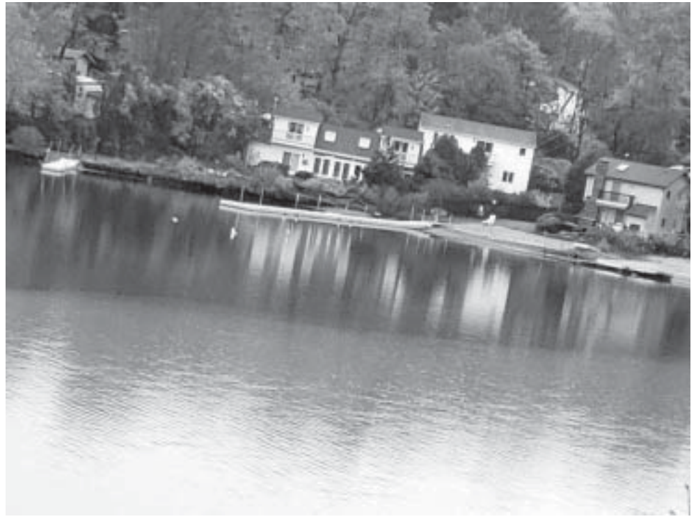
East Hampton Planning and Zoning Official Jeremy DeCarli said runoff from the $18.98 million municipal hub site on Route 66 is responsible for a large area of sediment deposited in the back bay of Lake Pocotopaug last month. This contributed photo shows the cloudy sediment in the foreground.
