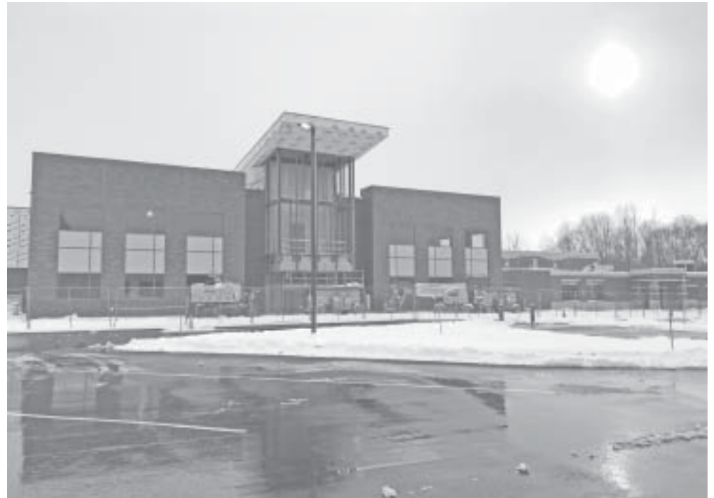
The face of the new William J. Johnston Middle School in Colchester will feature an enclave of glass, shown above – which will be used by eighth grade students as a gathering space.
