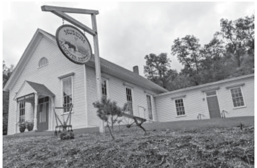
After several months of searching for a contractor to replace the lower roof on the Andover Museum, the Board of Selectmen has hired Seacoast Construction. The museum holds items with significance to local history, such as coal stoves, looms, spinning wheels, a carriage, a sleigh, postcards and photos and has a large mural painted by local artists depicting major events in Andover history from the 1600s to now.
